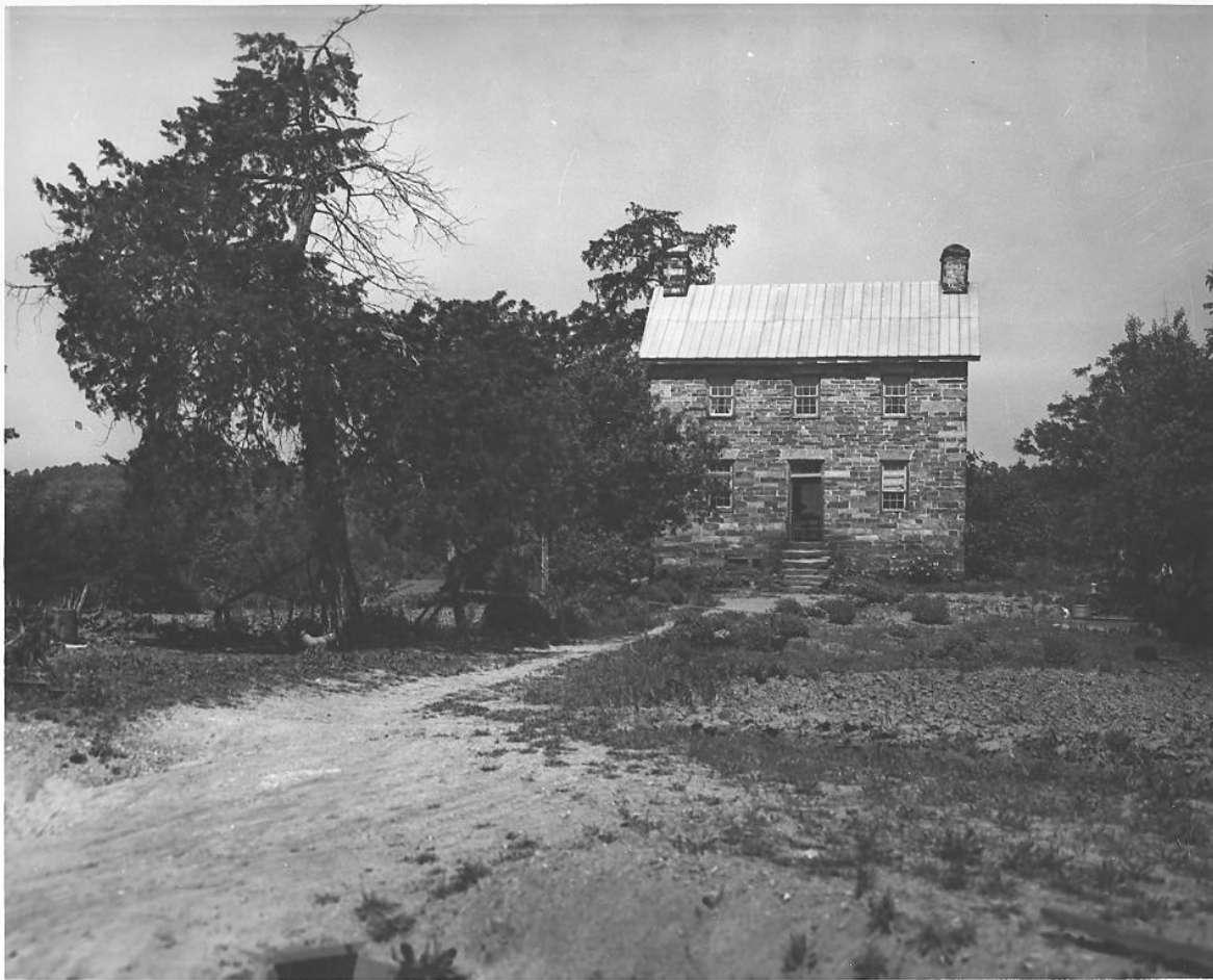
Figure 4. Historic image of Henry Howser House (built approximately 1803). Howser was a stone mason and built his house from local stone quarried within the park. NPS Photo courtesy Chris Revels (NPS Kings Mountain NMP).
